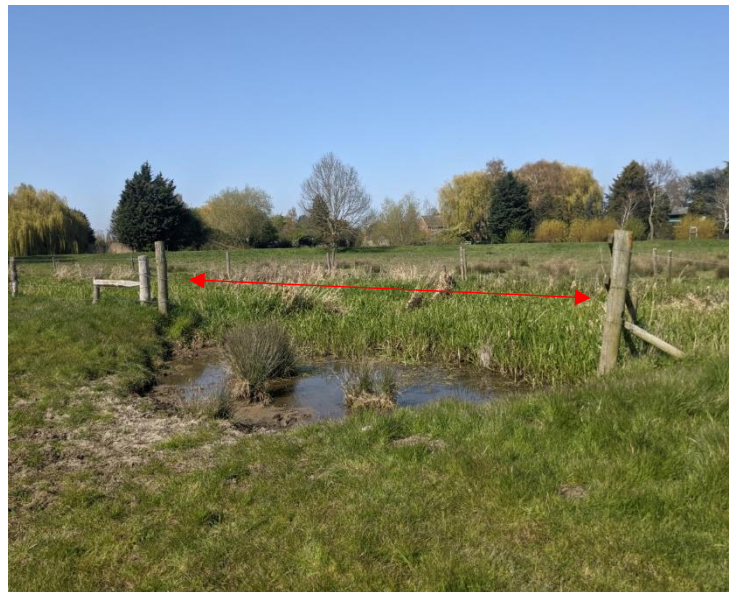
Fencing to be installed to block open gap.
