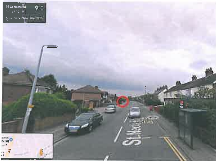
Image 3 - St Neots Road, South Bound. Existing shelter North Bound stop circled in red on image.
