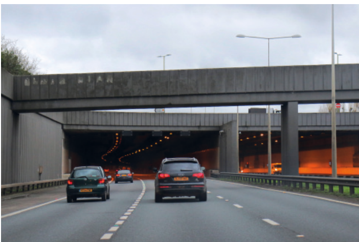
Photograph 5: Junction 3-4, motorway section
