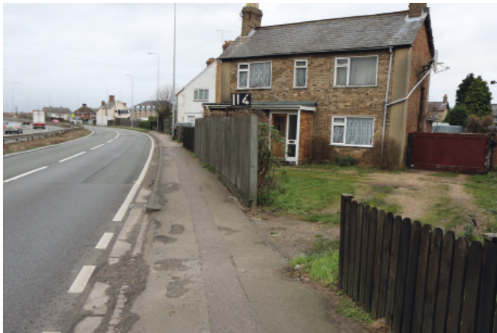
Photograph 8 - Sandy - Black Cat Roundabout. Poor townscape, poor quality footways and hazardous vehicular accesses.
